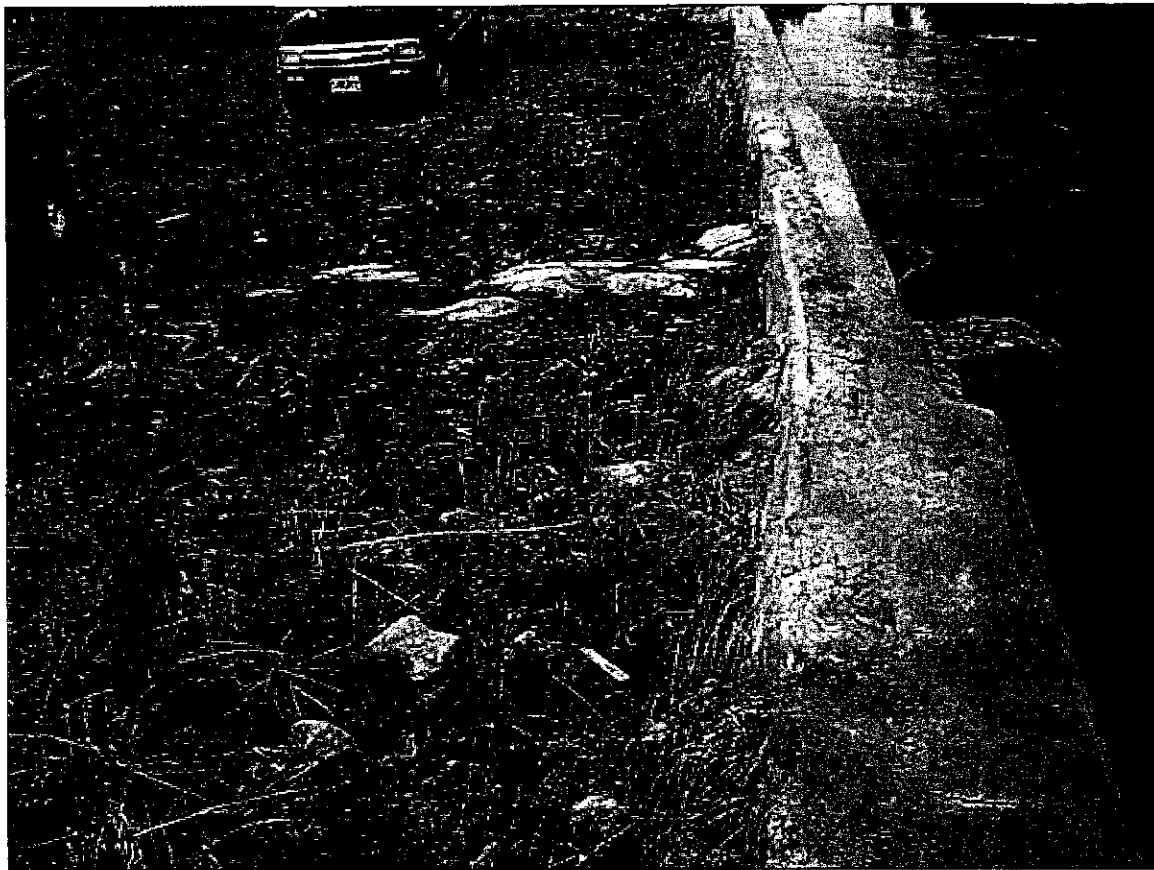
Leakage through canal wall near intake
