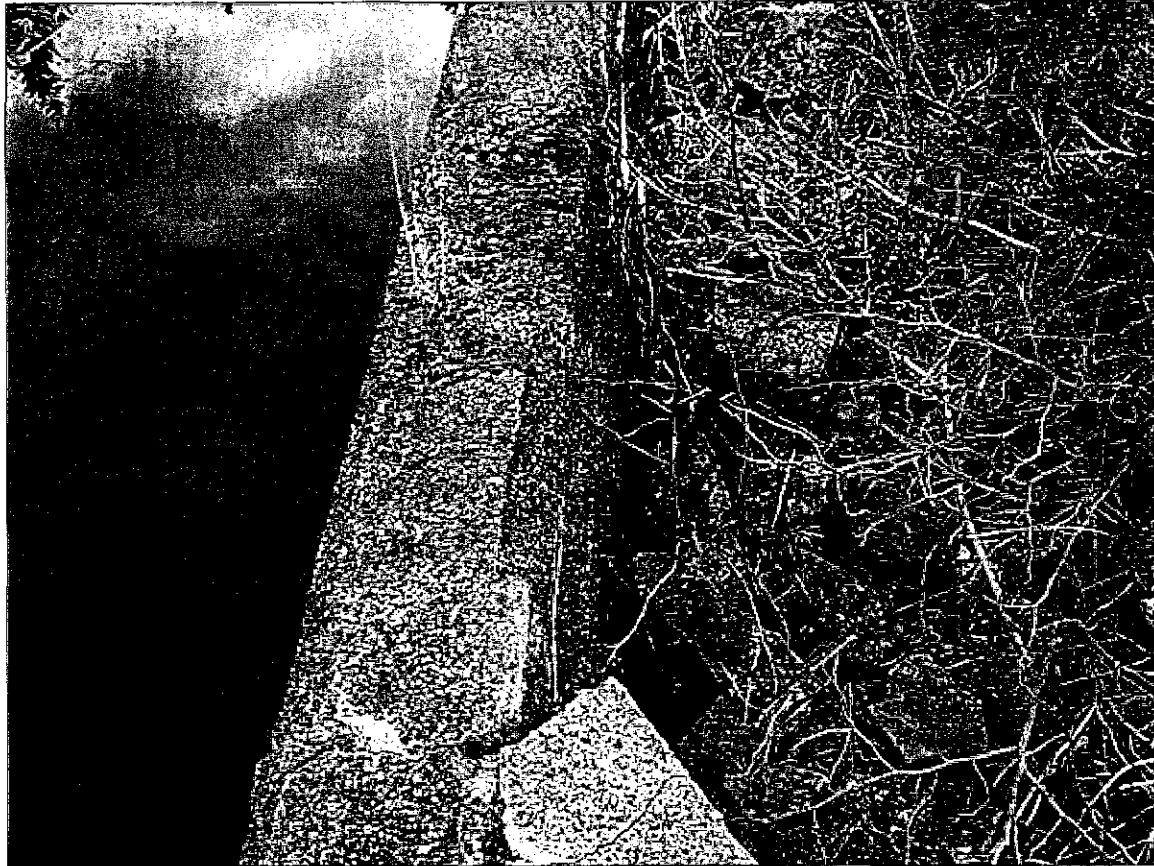
Concrete deterioration along canal walls
