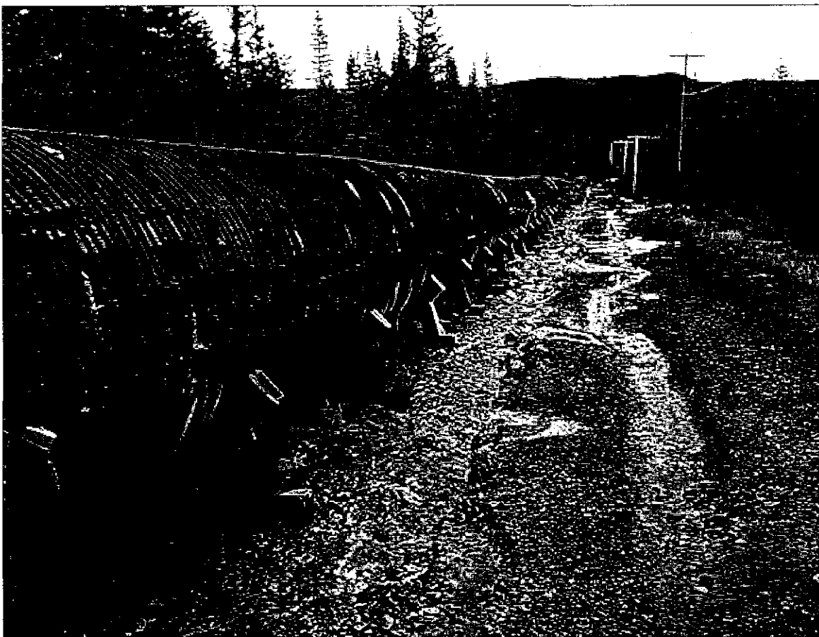
Looking downstream showing leakage along bedding and access road
